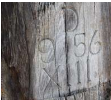
Original numbered carvings on timber bridge piers
