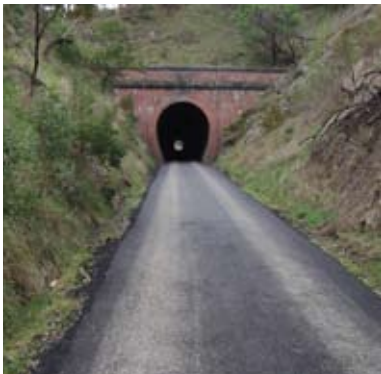
Cheviot Tunnel after track sealing
