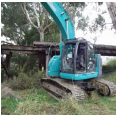
Removing bridge deck timbers
