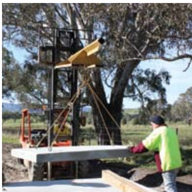
Loading concrete decks
